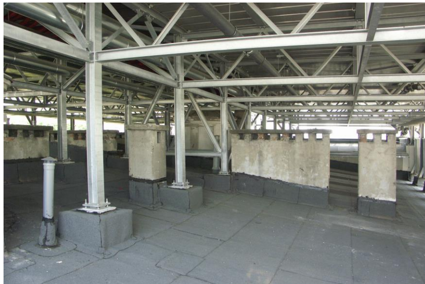
Figure 3. The steel structure of the hospital helipads on Lindley Street in Warsaw
